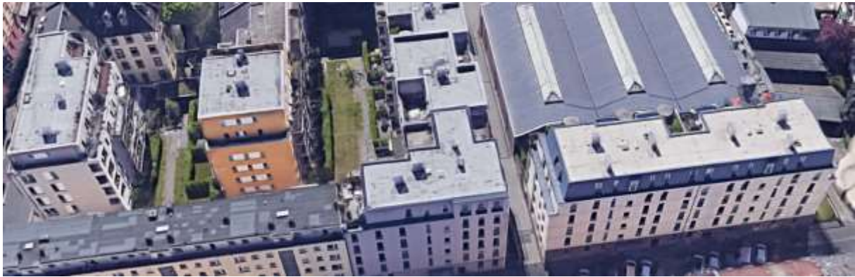
Figure 98: View of new buildings
