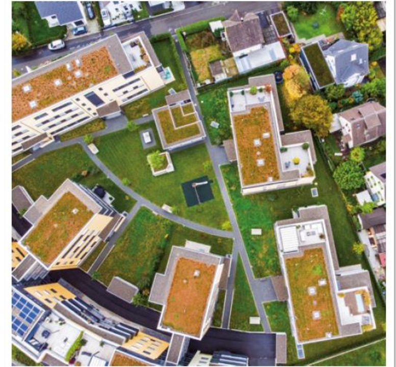
Fig.: Green rooftops © Heiner / stock.adobe.com
