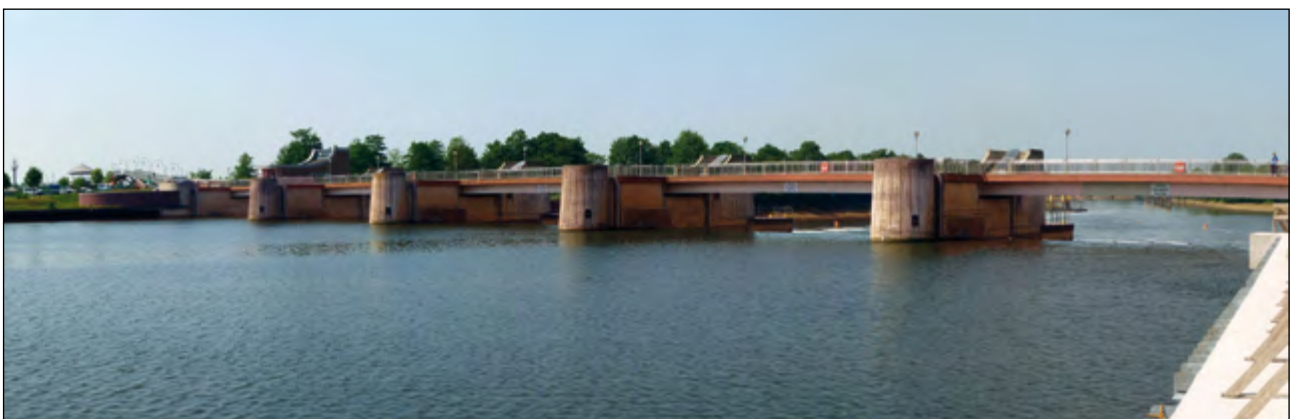
Figure 66: Barrage weir for hydropower generation in Bremen-Hemelingen
