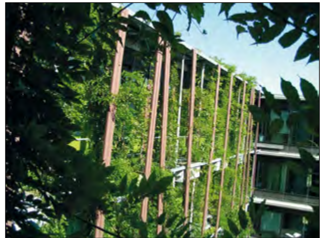
Figure 45: Facade planting in the courtyard of the Institute of Physics at Humboldt University, Berlin-Adlershof
