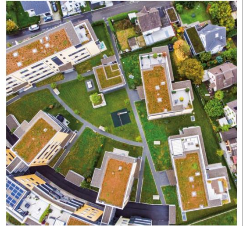
Fig.: Green rooftops © Heiner / stock.adobe.com
